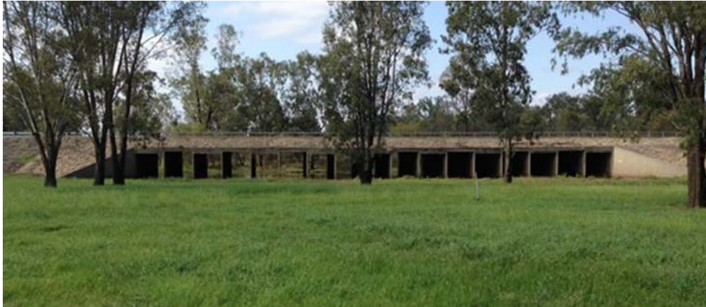
Figure 3.4 DAWSON RIVER OVERFLOW CULVERTS AT LEICHHARDT HWY, TAROOM
