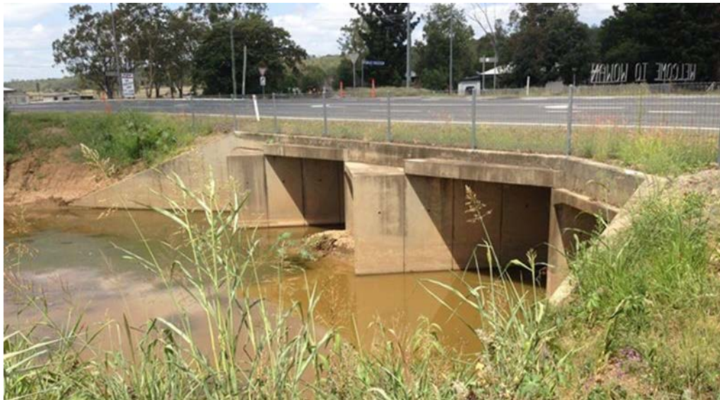
Figure 3.5 POCKET CREEK CULVERTS UNDER LEICHHARDT HWY, WOWAN
