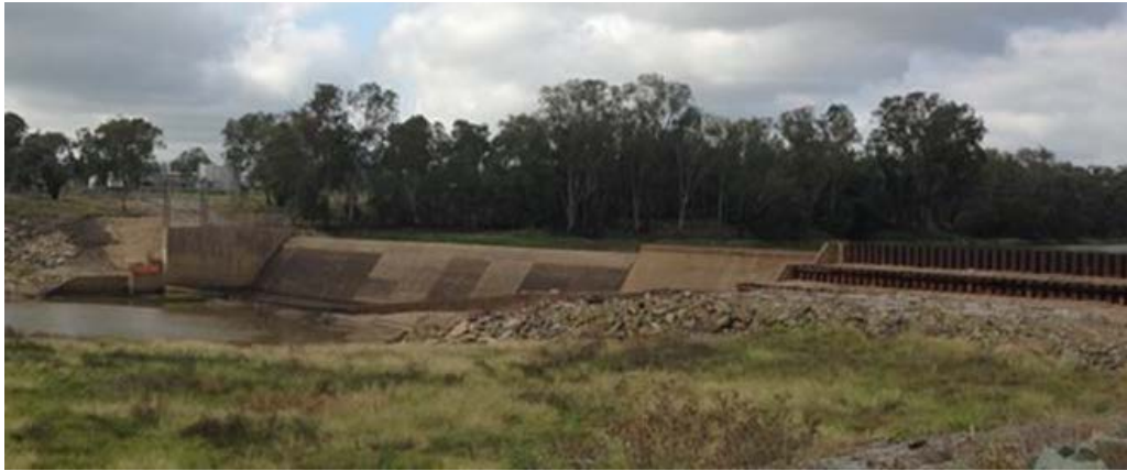
Figure 3.2 NEVILLE HEWITT WEIR ON THE DAWSON RIVER AT BARALABA
