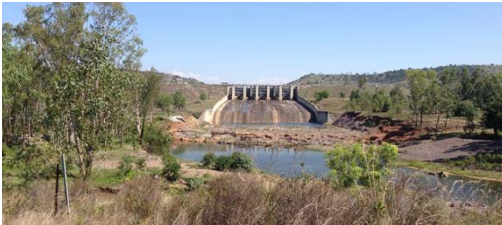
Figure 3.3 CALLIDE DAM SPILLWAY NEAR BILOELA
