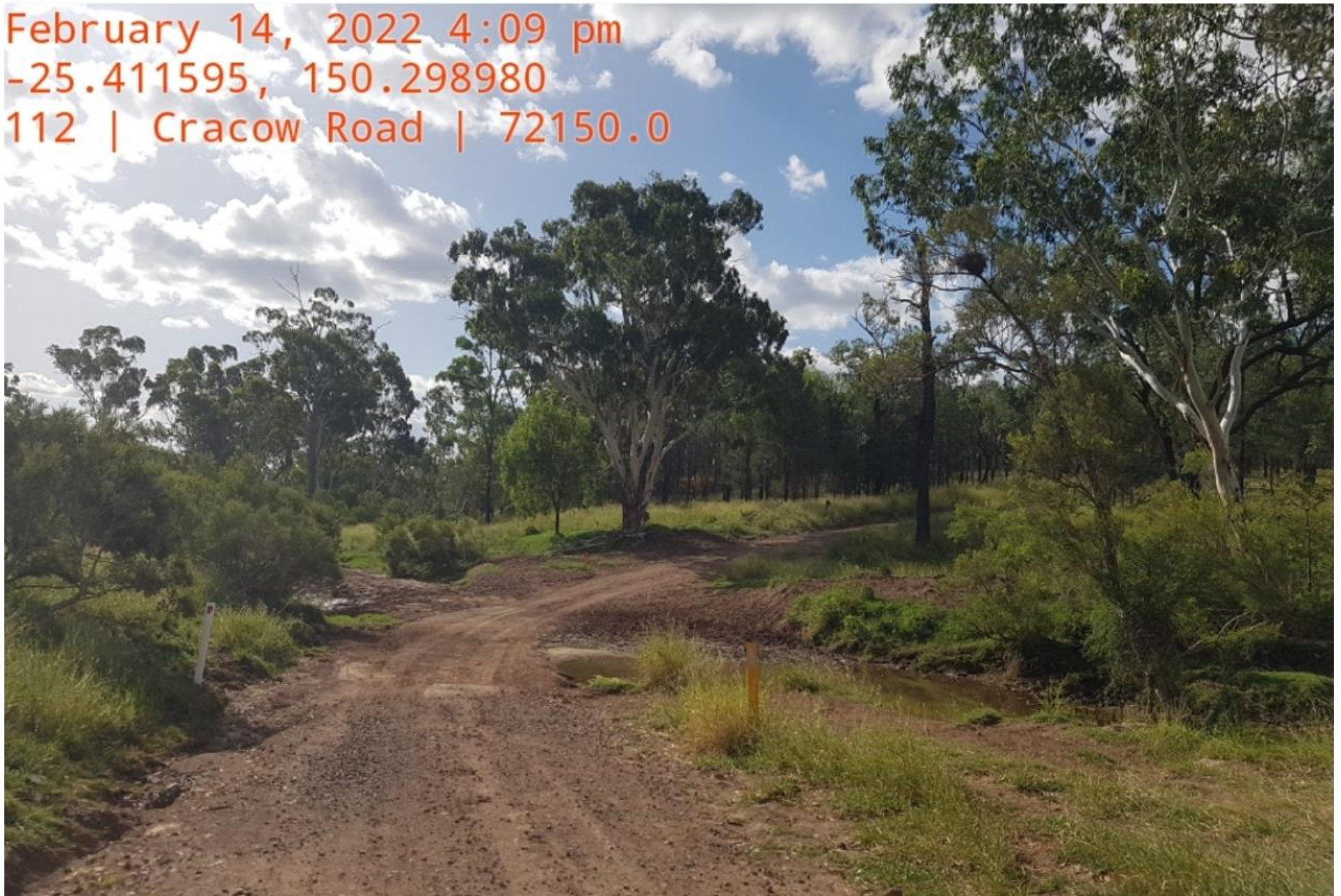
Ross Creek CH72200 Replace existing creek bed level concrete floodway
