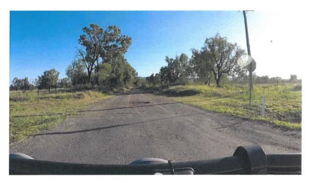
Figure 4-1 - Shorts Road Ch-02 - Biloela, QLD (Fatigue cracking above culvert - Sealed intersection)
