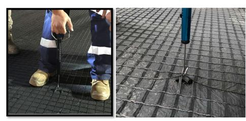
Reference images showing adequate bond following installation onto the tack-coated surface
