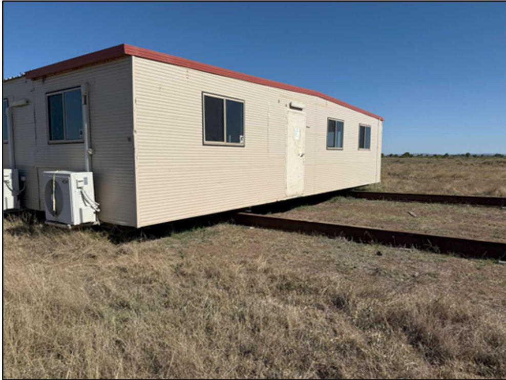
Figure 1 – Building on rails (source – Qantac)
